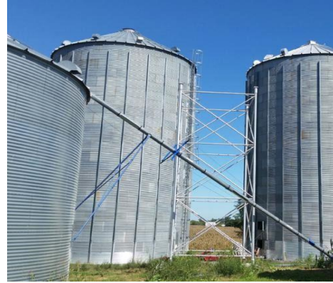
Figure : 19 Cement Bins
